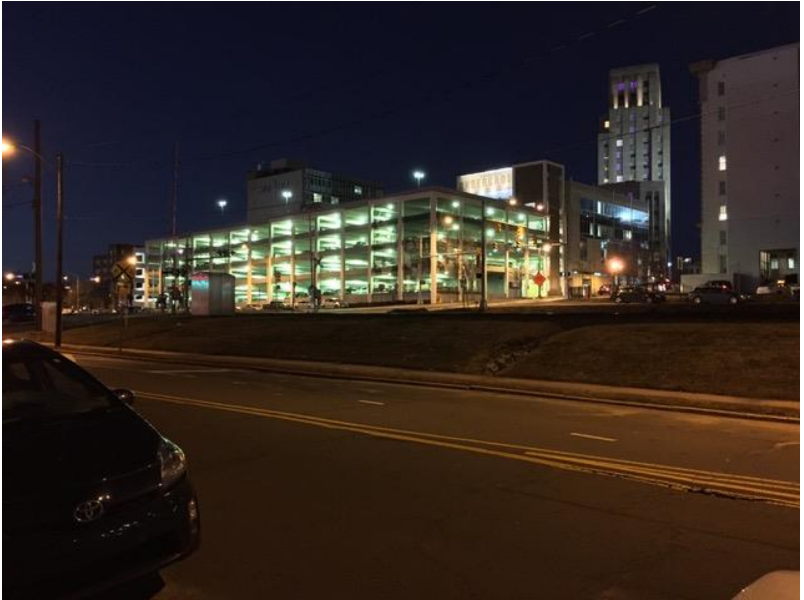
Corcoran Street Garage – Present Condition – Night View
